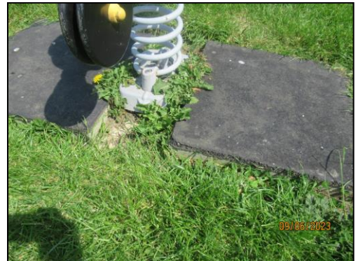
(Potential trip hazards at edges of tiles)
