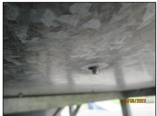
(Protruding rivets)
