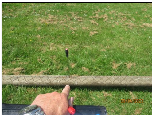
(Rotten incline balance beam)
